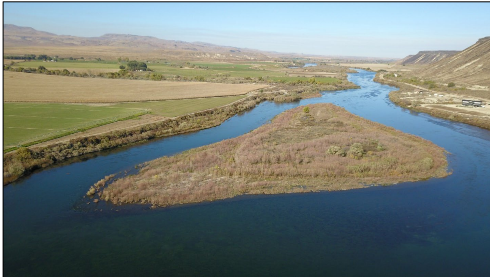
Bayha Island expansion four years post construction, Snake River, ID.
