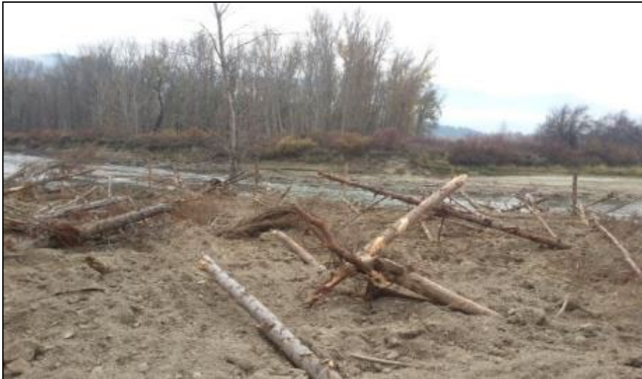
Example floodplain roughness post-construction.
