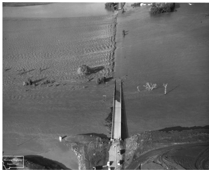
Flooding on Marias River near Shelby, MT, June 1964. Photo by Montana Highway Department.
