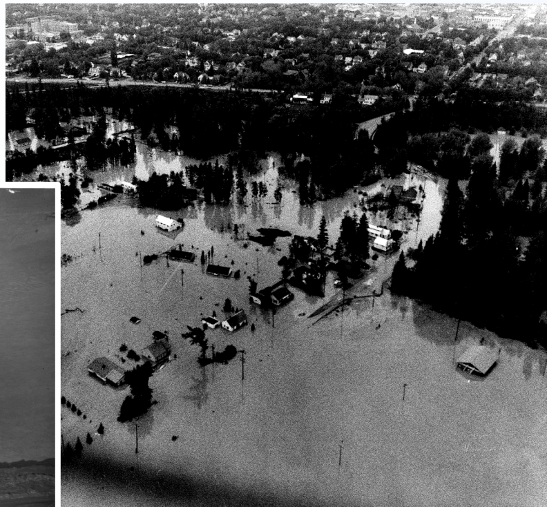
Flooding of Woodland Park, east side of Kalispell, June 1964. Photo by Guest Photo.
