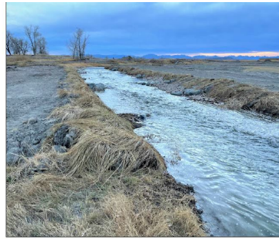
EXAMPLE PHOTO OF A GRADE CONTROL RIFFLE INSTALLED FOR SCHOOL SECTION, PHASE 1
