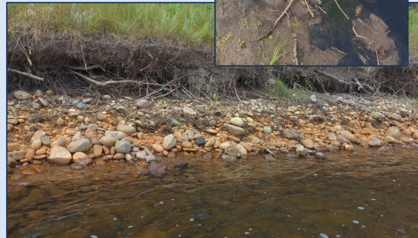
Iron and manganese staining
